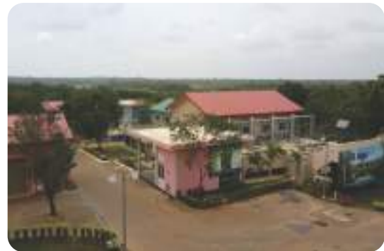
water treatment plant at Ruhunupura WSP
