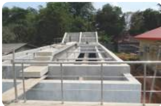
Water Treatment Plant in Mahiyanganaya
