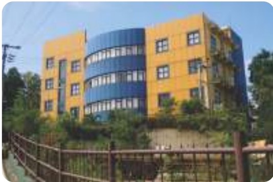
Regional Support Center Building at Kadawatha
