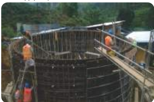
Construction of wash water recovery tank
