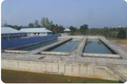
Completed sedimentation tanks and collecting channels
