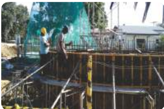
Tower construction at Velanai
