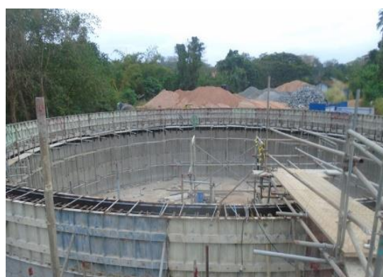
Construction of Sedimentation Tanks
