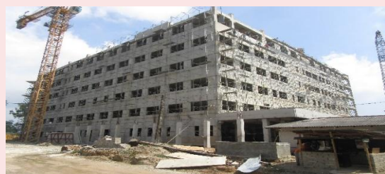
Construction works of Maternity Hospital, Galle
